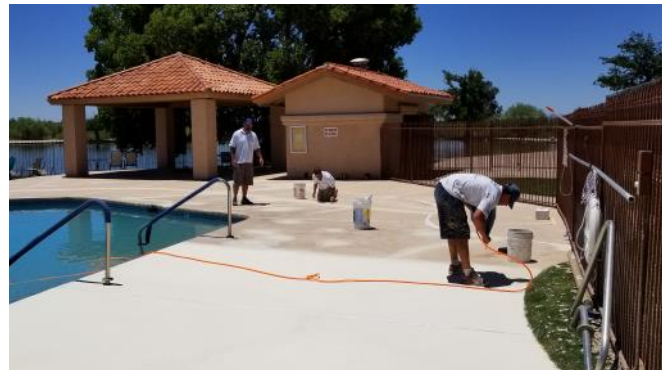
Deck resurfacing at Rec Center Pool
